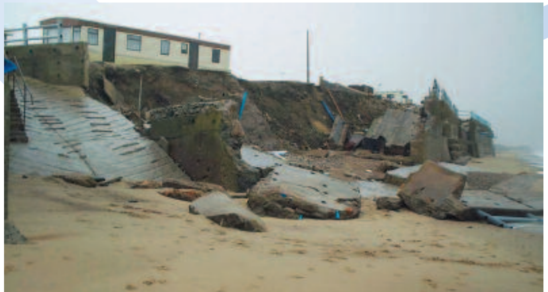
Failure of private defences at Ulrome, spring 2004
