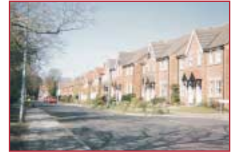
Ings Lane. Built 1980 - 90.
