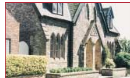
30/32 Station Road. Previously the National School.
