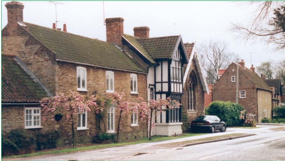
Para 7.3 Mix of Building Styles - Church Street
