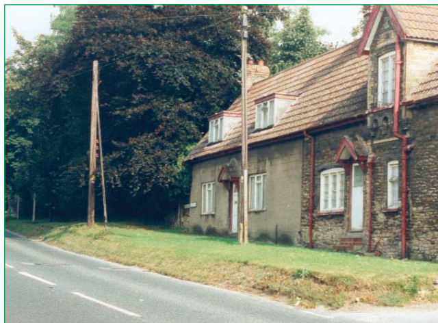
Para 5.15 Grass Verges - Station Road
