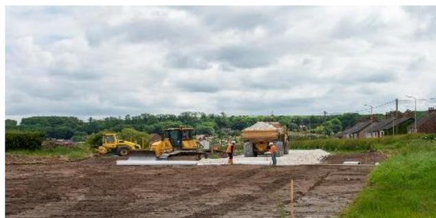
*Footprint of embankment stripped of topsoil and stone haul road being installed at South Ferriby*
